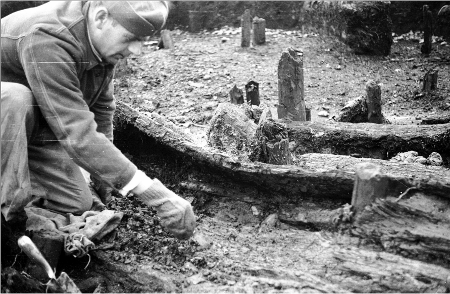
Fig. 13. Excavations at Pfyn-Breitenloo. Polish soldier at work. Photo from the archive Amt für Archäologie Thurgau.
