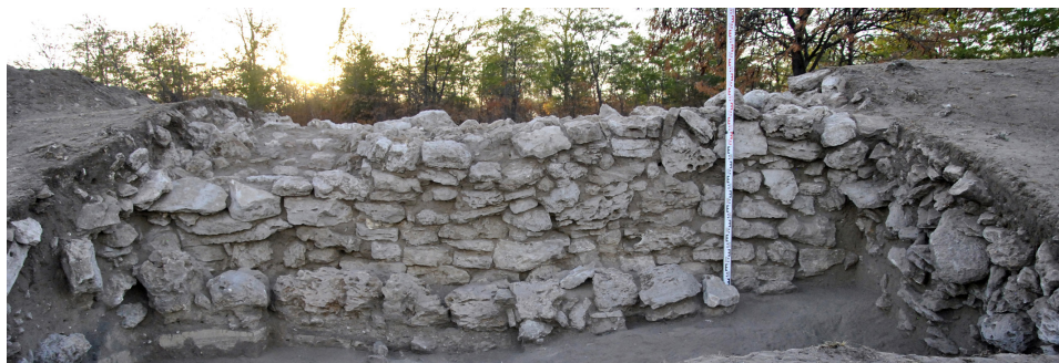
Fig. 7. Eastern facade of defensive wall and a stone buttress discovered in Trench II. Photo: M. Matera.
