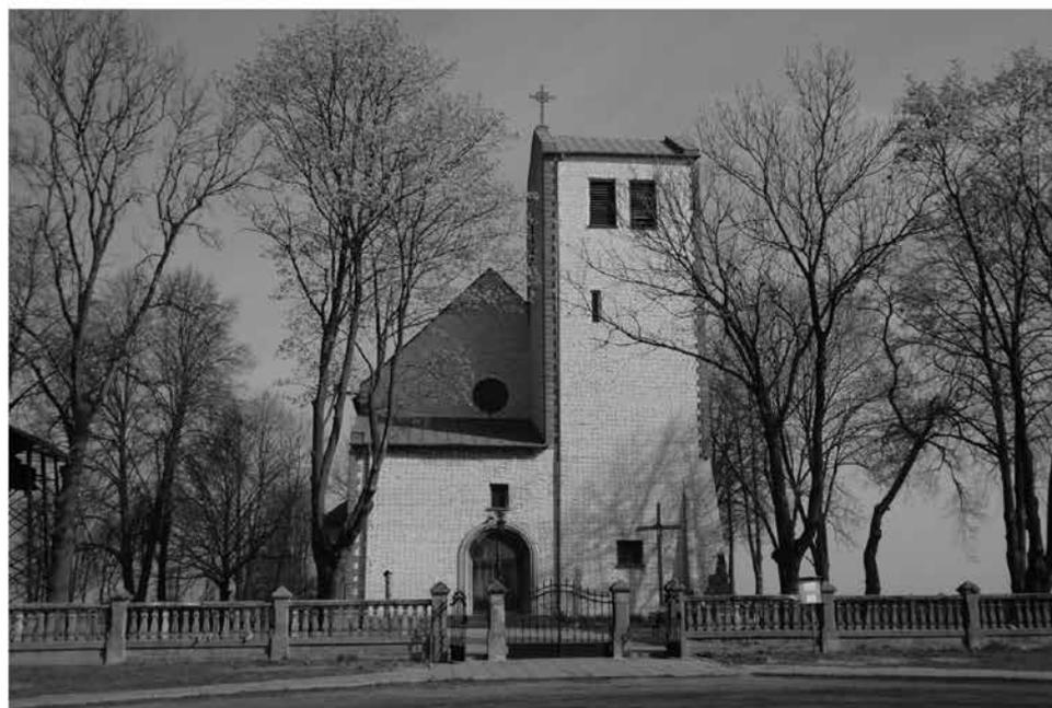
Fig. 3. Structures built of calcareous marl. Sobótka, Poddębice district (a), Wilamów, Poddębice district (b).
