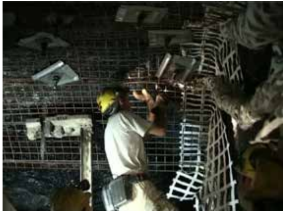
Tunnel reinforcement, in the Monte Sinni Nuraxi Figus coal mine, 2007
