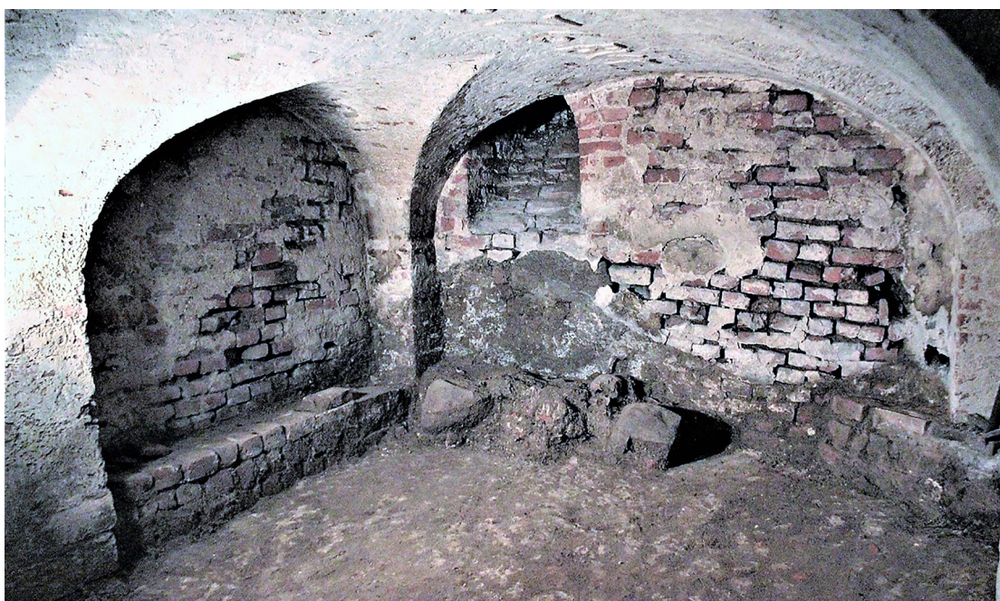
Fig. 17. Piaseczno. Original level of the crypt discovered after removing coffins, garbage and soil. Photo D. Grupa.
