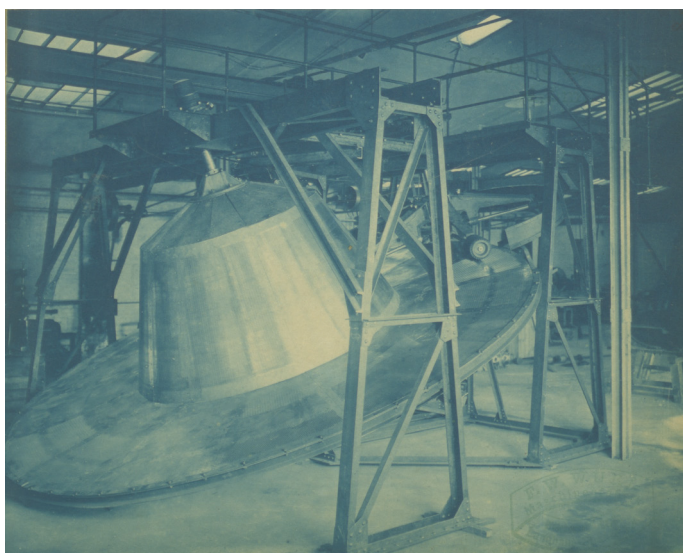
Fig. 9. Riensch Wurl system separator for sewage treatment plant Lower Wik/Dolny Wik (Unterwiek), 1914. Source: APS, AMS III/1302.
