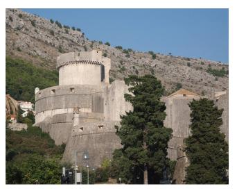
Fig. 17. Dubrovnik (Croatia). Minčeta tower and surrounding outer wall and curtain rebuilt by Michelozzo from 1461.
