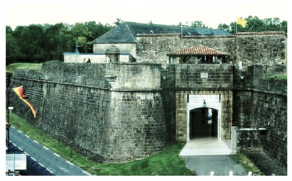
Fig. 20. Navarrenx (Pyrénées Atlantiques), bastion fortress built by Italian engineer 1530s. Photo P. Purton.
