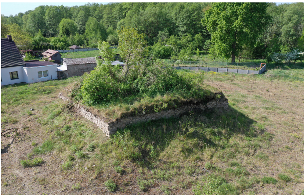
Fig. 8. Relics of the stone tower after the demolition of the site. East view taken in 2022. Photo: H. Augustyniak.
