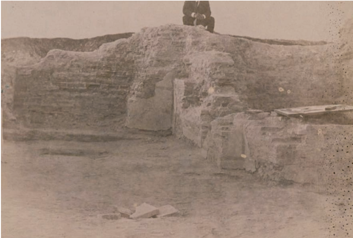
Fig. 14. The foundations of the church – “Old Cathedral”. Photo by A. Prakhov 1986. Photo provided in Album... 1889
