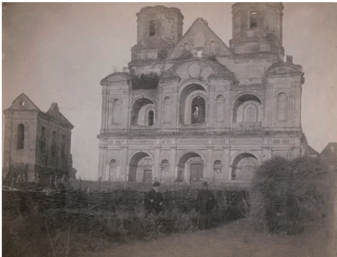
Fig. 6. View of the Assumption Cathedral in Volodymyr-Volynskyi from the southwest. Photo by A. Prakhov 1986. Photo provided in Album... 1889
