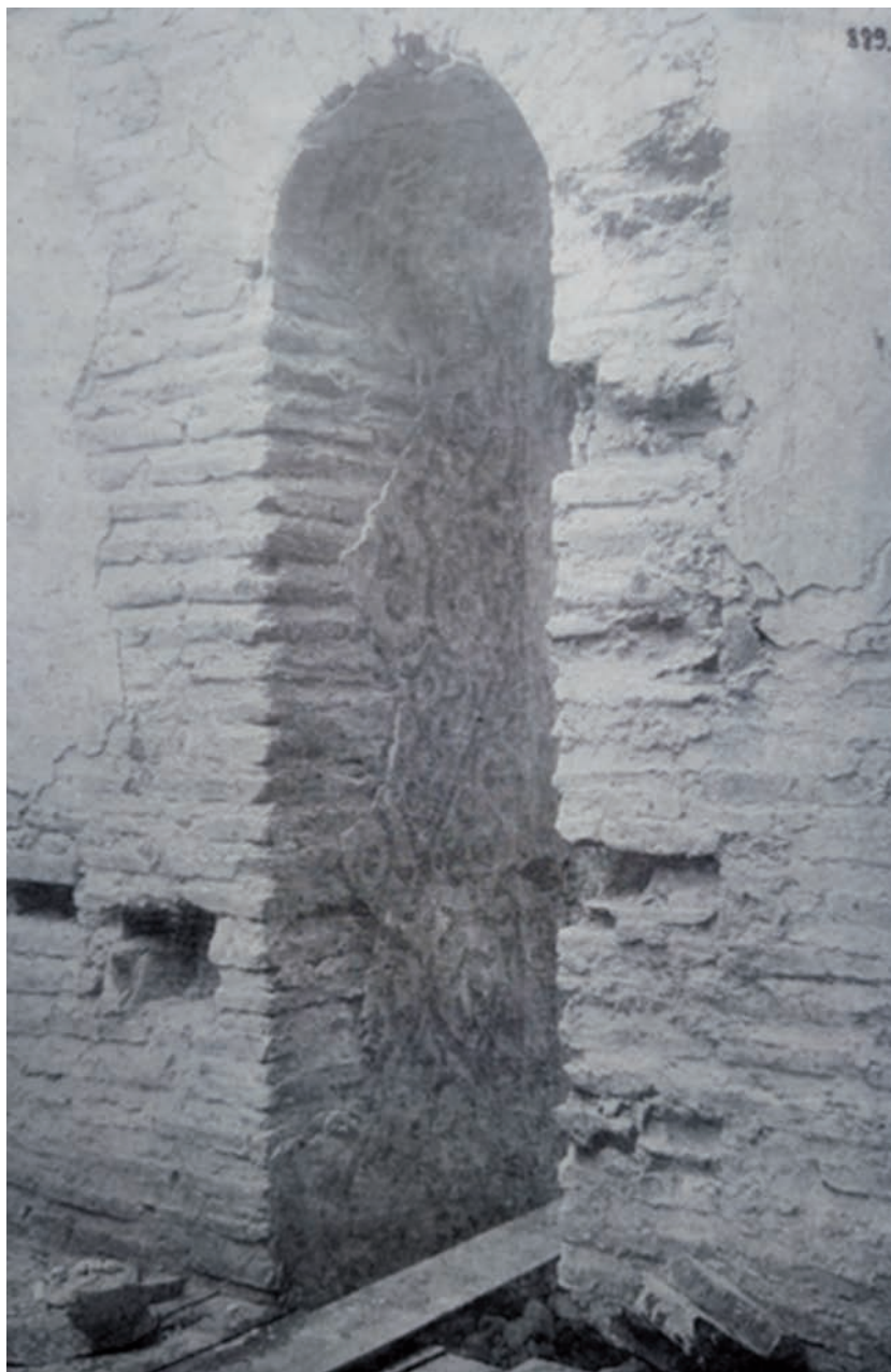
Fig. 11. Window hole with frescoes in the Assumption Cathedral. Photo of 1897. Photo provided in Rappoport 1977
