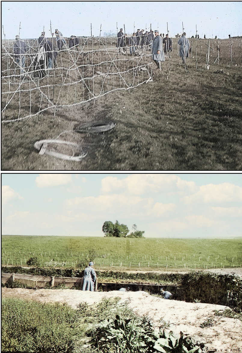
Fig. 11. Examples of passive anti-personnel obstacles: upper panel – Kraków area. The photograph of an Austro-Hungarian anti-personnel obstacles made from barbed wire and plain wire in the foreground of the position from 1914. Note that the picture shows a roll of plain wire, analogous to the item discovered at the Raciborowice-Prawda, Site 3. Österreichische Nationalbibliothek, Wien, ref. no Pk 5090, 42, colourised by K. Przybysz-Malczewski, lower panel – Lytovezh, Volyn Oblast (Ukraine). The photograph of an Austro-Hungarian fortified position from First World War in an elevated area with the foreground secured with wire obstacles, analogous to the position discovered at the Raciborowice-Prawda, Site 3.
