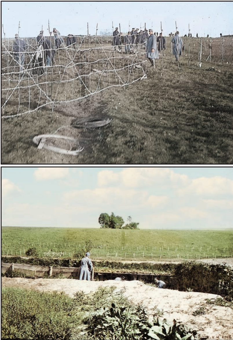
Fig. 11. Examples of passive anti-personnel obstacles: upper panel – Kraków area. The photograph of an Austro-Hungarian anti-personnel obstacles made from barbed wire and plain wire in the foreground of the position from 1914. Note that the picture shows a roll of plain wire, analogous to the item discovered at the Raciborowice-Prawda, Site 3. Österreichische Nationalbibliothek, Wien, ref. no Pk 5090, 42, coloured by K. Przybysz-Malczewski, lower panel – Lytovezh, Volyn Oblast (Ukraine). The photograph of an Austro-Hungarian fortified position from First World War in an elevated area with the foreground secured with wire obstacles, analogous to the position discovered at the Raciborowice-Prawda, Site 3.
